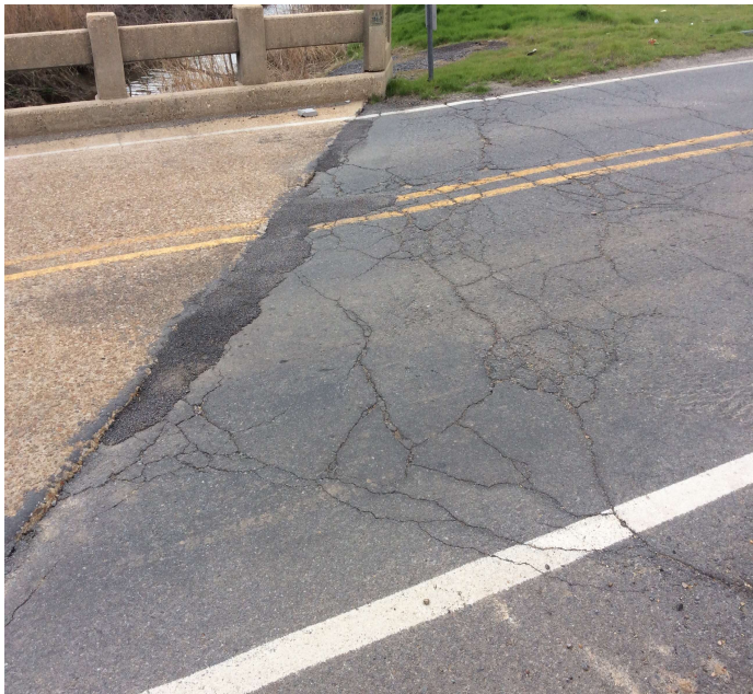
PHOTO 1 Description Approach roadway - Bent 1 (deterioration)
