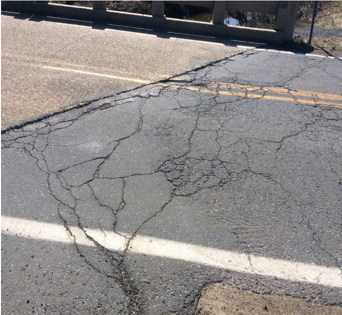
PHOTO 3 Description Bent 1 - Approach Roadway: Deterioration/settlement
