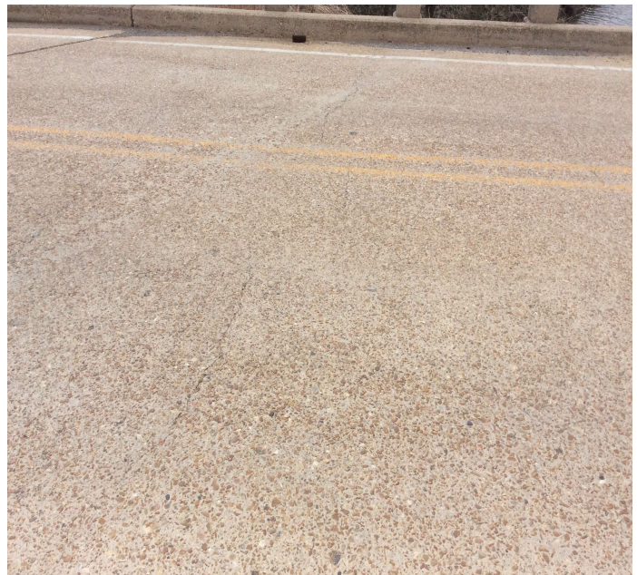
PHOTO 2 Description Deck - Span 2 (cracking)
