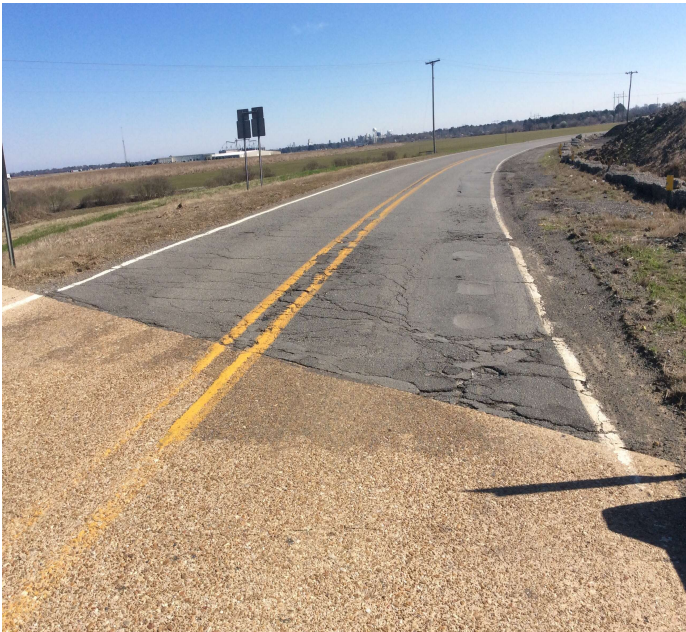
PHOTO 4 Description Bent 4 - Approach Roadway: Deterioration
